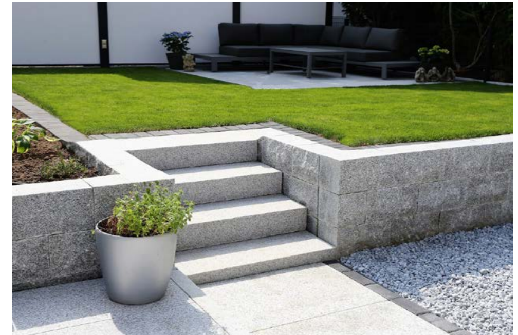
Example - steps incorporated within the lower private amenity space to help minimise cut/fill. In places, wider steps can be incorporated and utilised as informal places to sit
