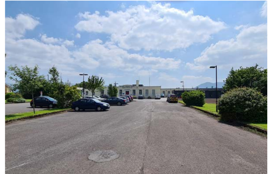
View 3 - Killarney Community Hospital to the north of the Site
